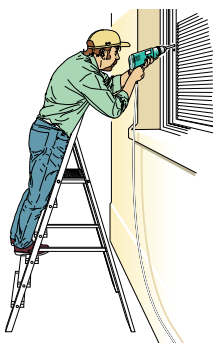
Figure 2b Correct - steps facing work activity
