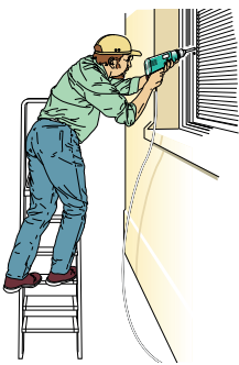
Figure 2a Incorrect - steps side-on to work activity
